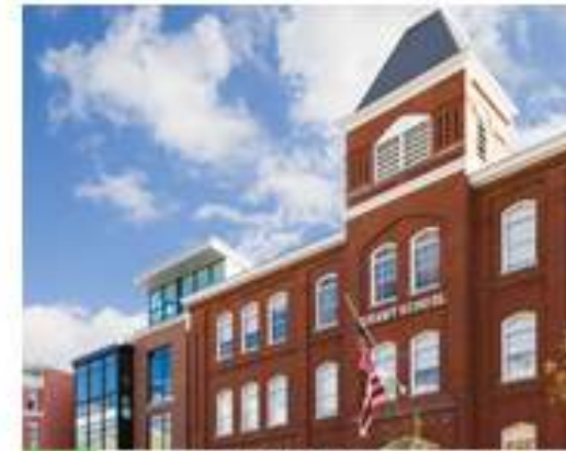
5 Defer to the Civic Presence of the Historic Structures
